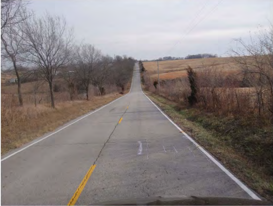
Photo 13 – View east along NE 112 th Street. NE 112 th Street is the northern border of the Redevelopment Area at this location. Additionally, NE 112 th Street has numerous locations with very limited sightlines and vehicular turning points.
