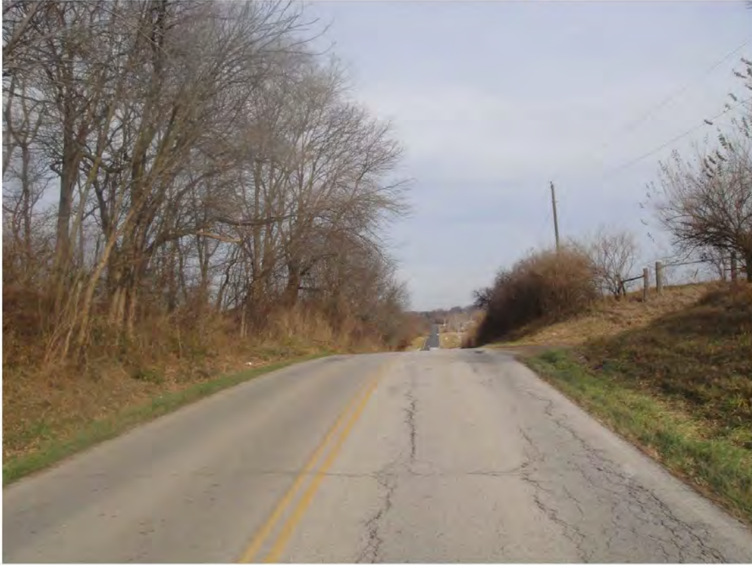
Photo 16 – View north along Plattsburg Road. Note limited sightlines and vehicular turning points.
