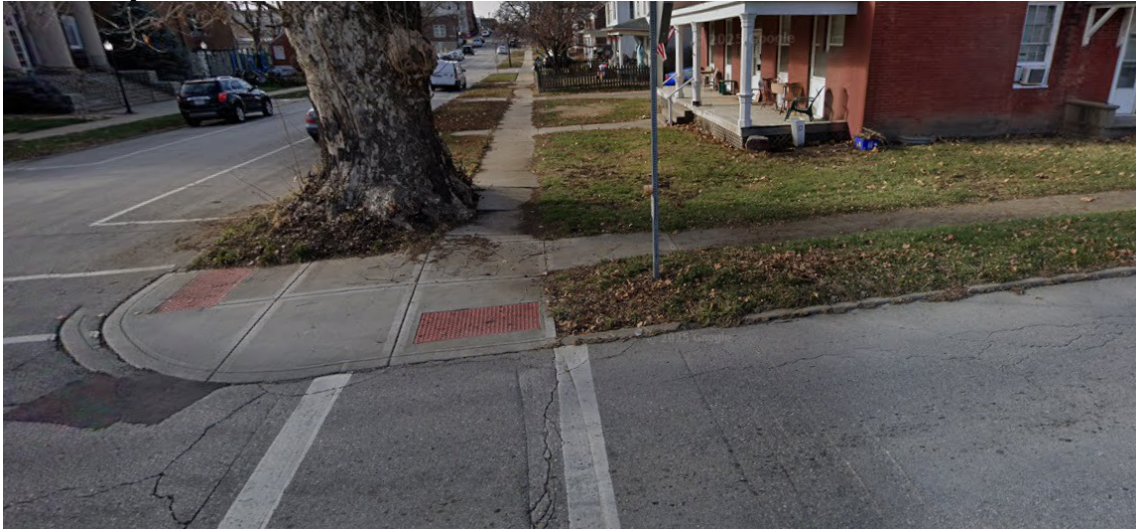
Figure 1 — Sidewalk and Tree Before Removal
