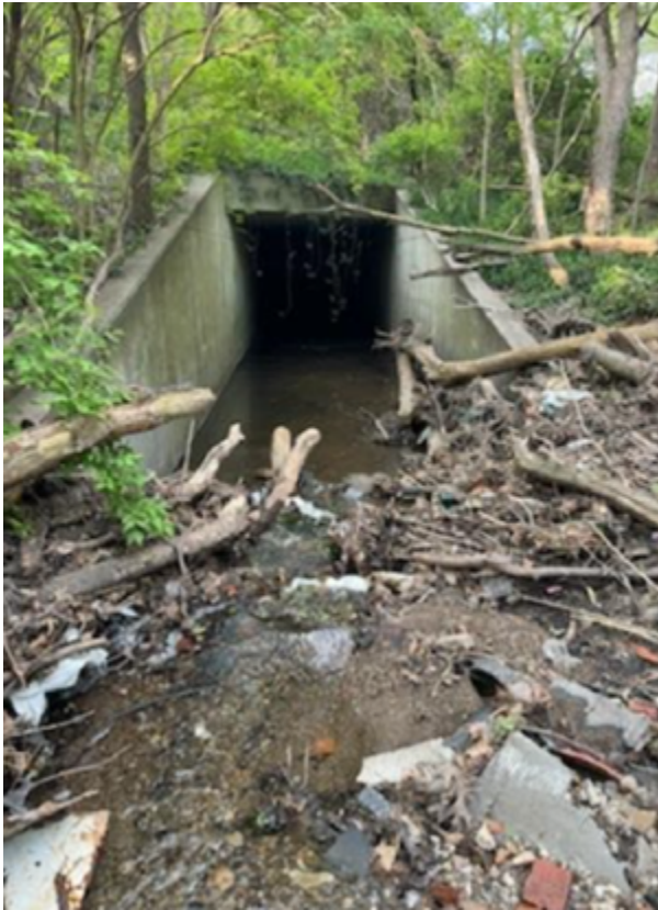
Figure 3 – Box Culvert Approach
