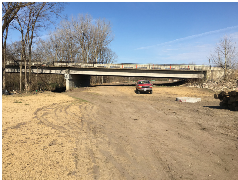
< Disturbance around the existing S Withers Rd overpass related to recent sewer improvements.
