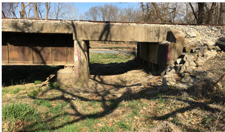
< The proposed railroad underpass location; clearance is approximately 8'-6".
