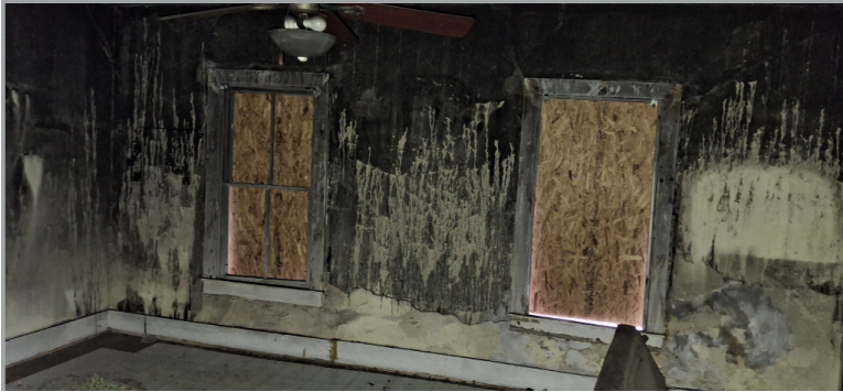
Front Bedroom Windows Existing Conditions
