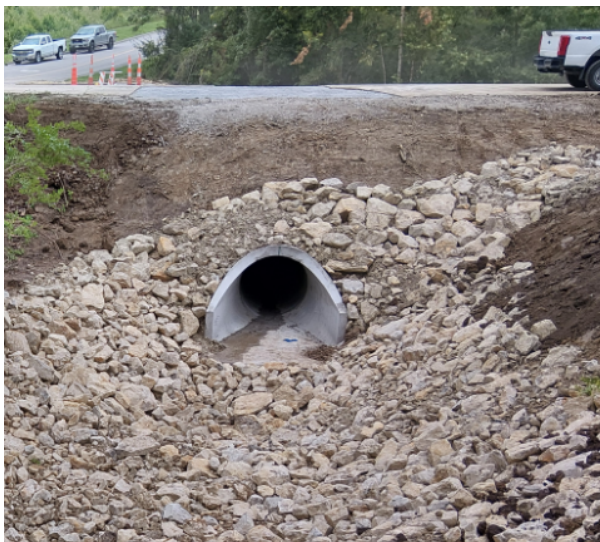
Figure 4 - 54" Reinforced Concrete Pipe Outfall
