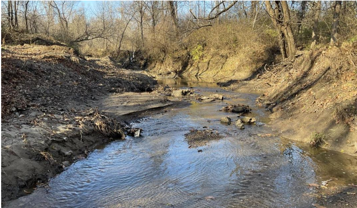
Figure 2-10. Stream bank erosion along Stream 9 (Location ID: S9.5)
