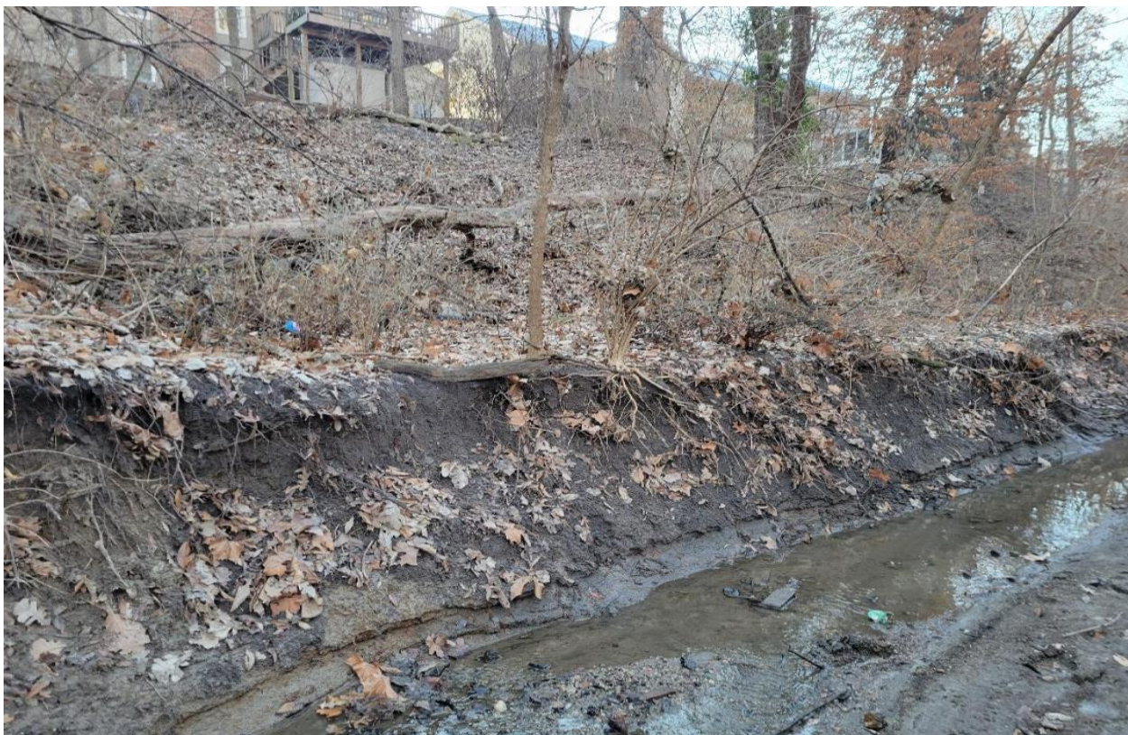
Figure 2-9. Stream Bank Erosion observed in Stream 8 (Location ID: S8.12)
