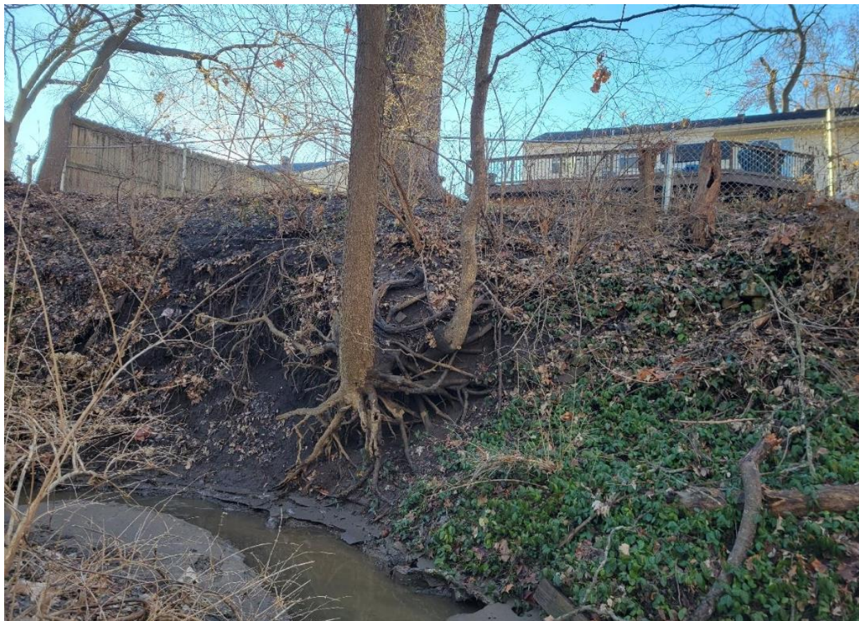
Figure 2-4. Observed Stream Bank Erosion along Stream 3 (Location ID: S3.24)
