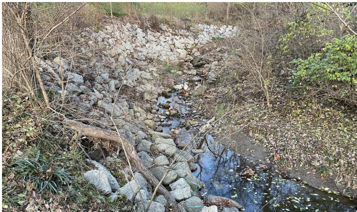
Figure 2-7. Rock Riprap along Bank on Stream 6 (Location ID: S6.23)
