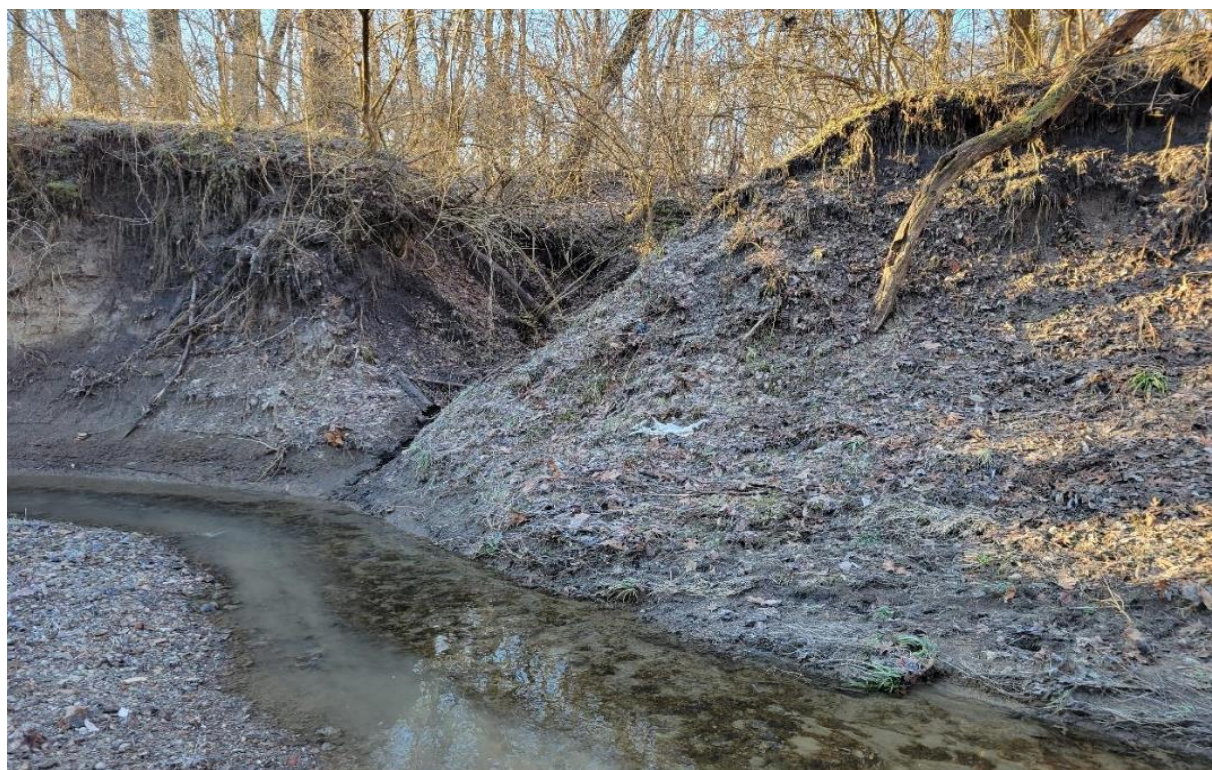
Figure 2-11. Stream Bank Erosion Observed along Stream 10 (Location ID: S10.3)
