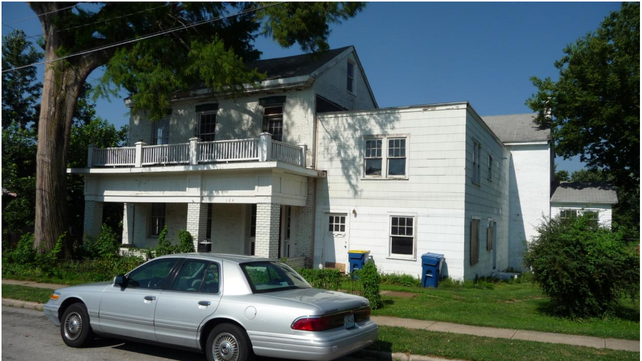
Physical Deterioration. 124 N. Gallatin. Historic home previously divided into apartments, but currently a single-family residence. Property has reported Nuisance Code Violations from lack of exterior maintenance. Social liability because it repeals other private local investment on surrounding properties.
