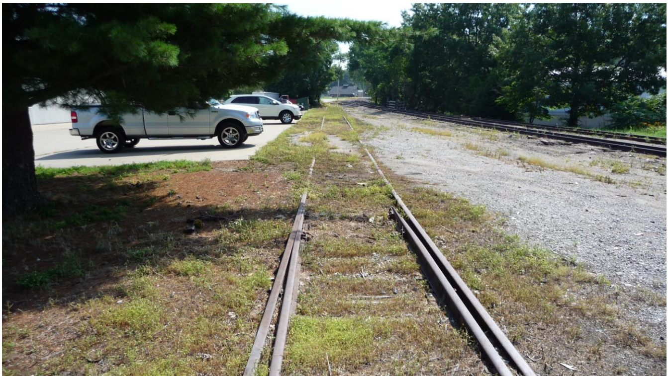
Obsolescence. Obsolete, unused rail spur. Possible trip and fall hazard due to overgrown rail lines.
