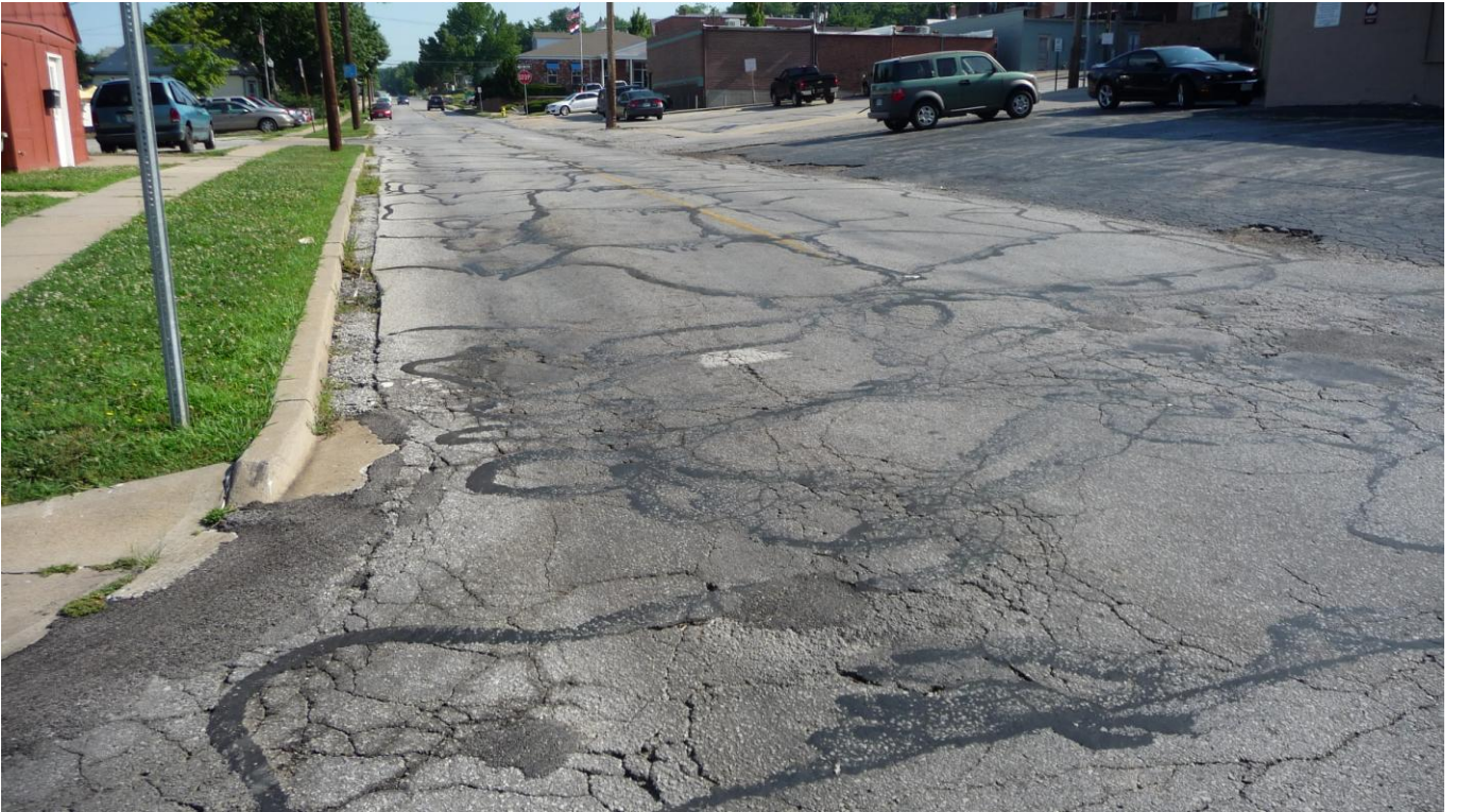
Physical Deterioration. Deteriorated pavement, curb & gutter. Social and economic liability, unattractive public access reduces likelihood of reinvestment.
