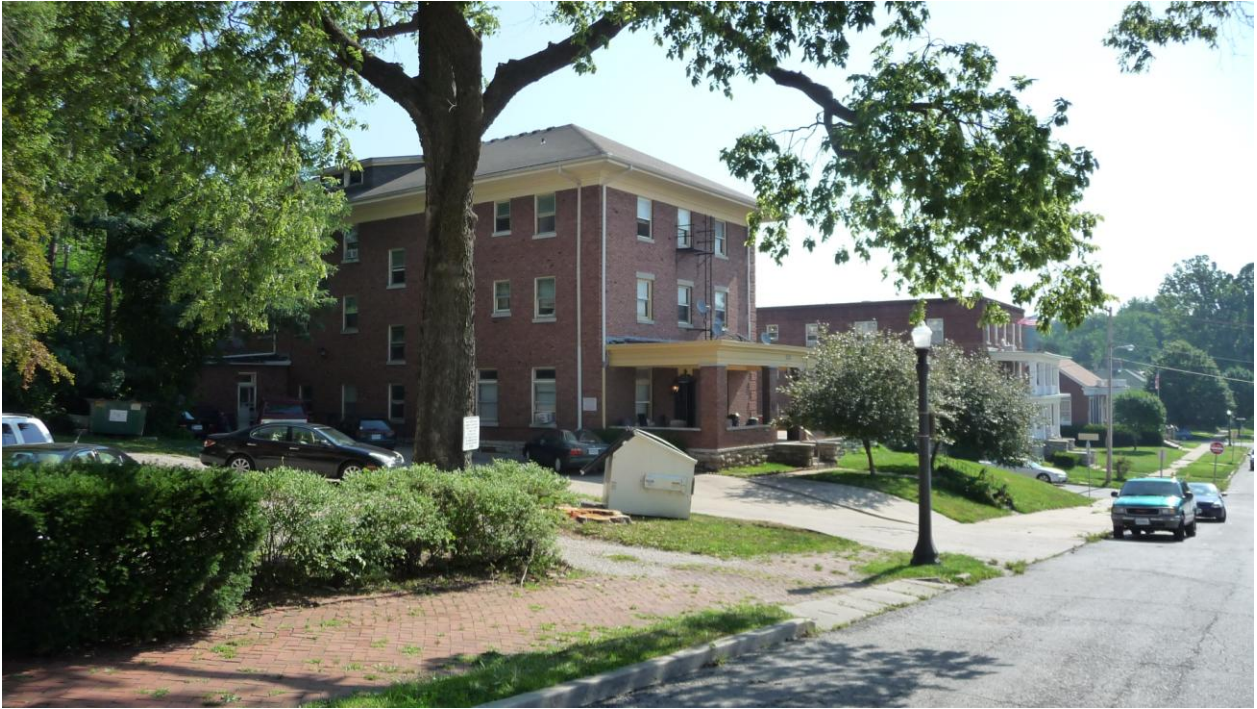
112 E. Franklin. Multi-family apartment building. Dumpster located in front yard is frequently reported as a Nuisance Code Violation due to scattered trash & debris overflowing around dumpster. Potential transmission of disease if trash not properly disposed of.
