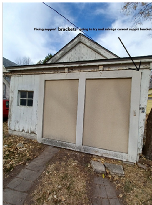
South Elevation of Garage
