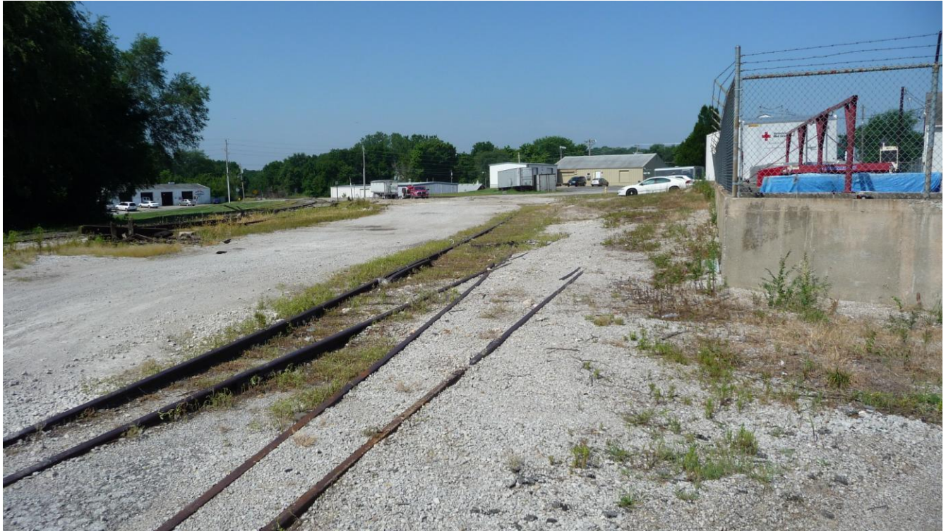
Obsolescence. Obsolete, unused rail spur. Overgrown weeds and scattered trash & debris. Economic liability due to unused nature of property.
