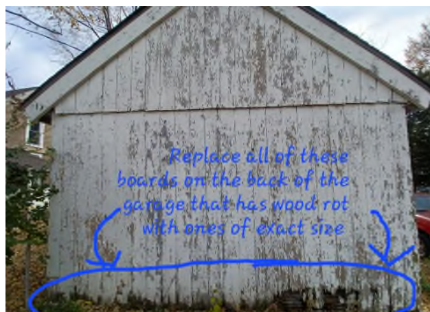
North Elevation of Garage
