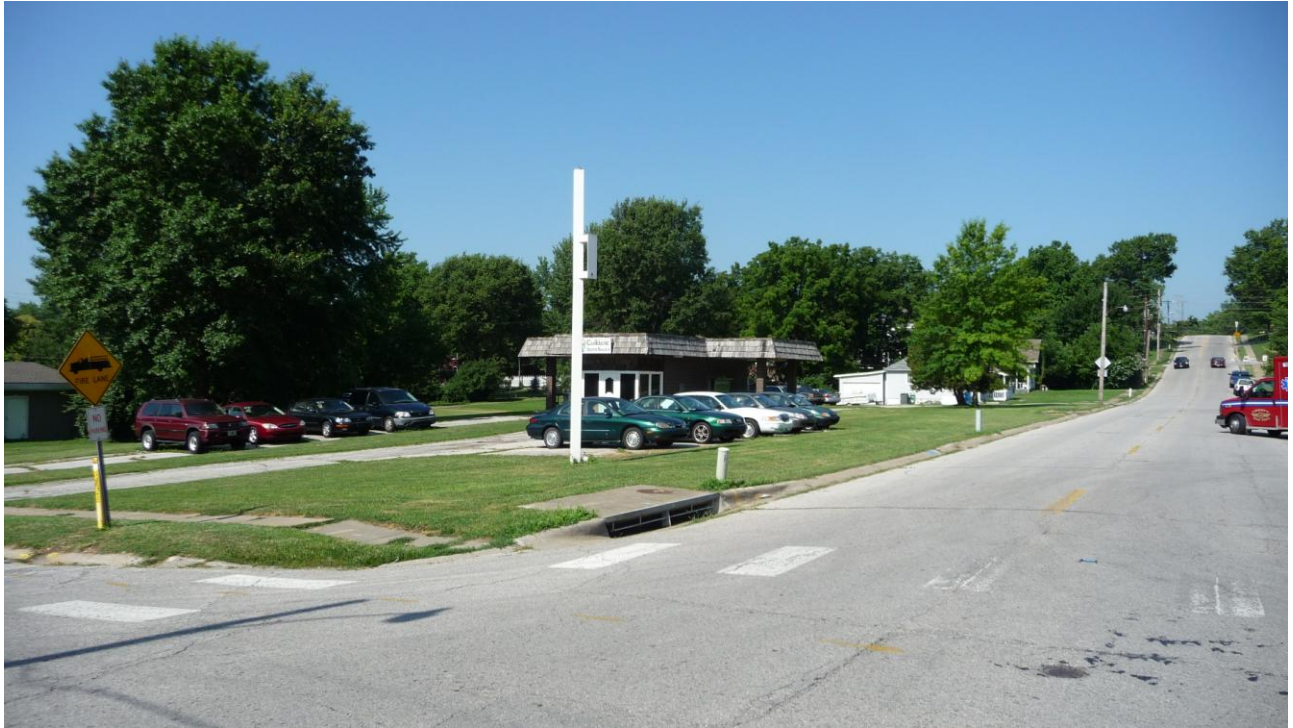
Obsolete Land Use. 201 West Mississippi. Former bank drive through now utilized as a used car and repair facility. Numerous Nuisance Code Violations for inoperable vehicles and other improper uses.
