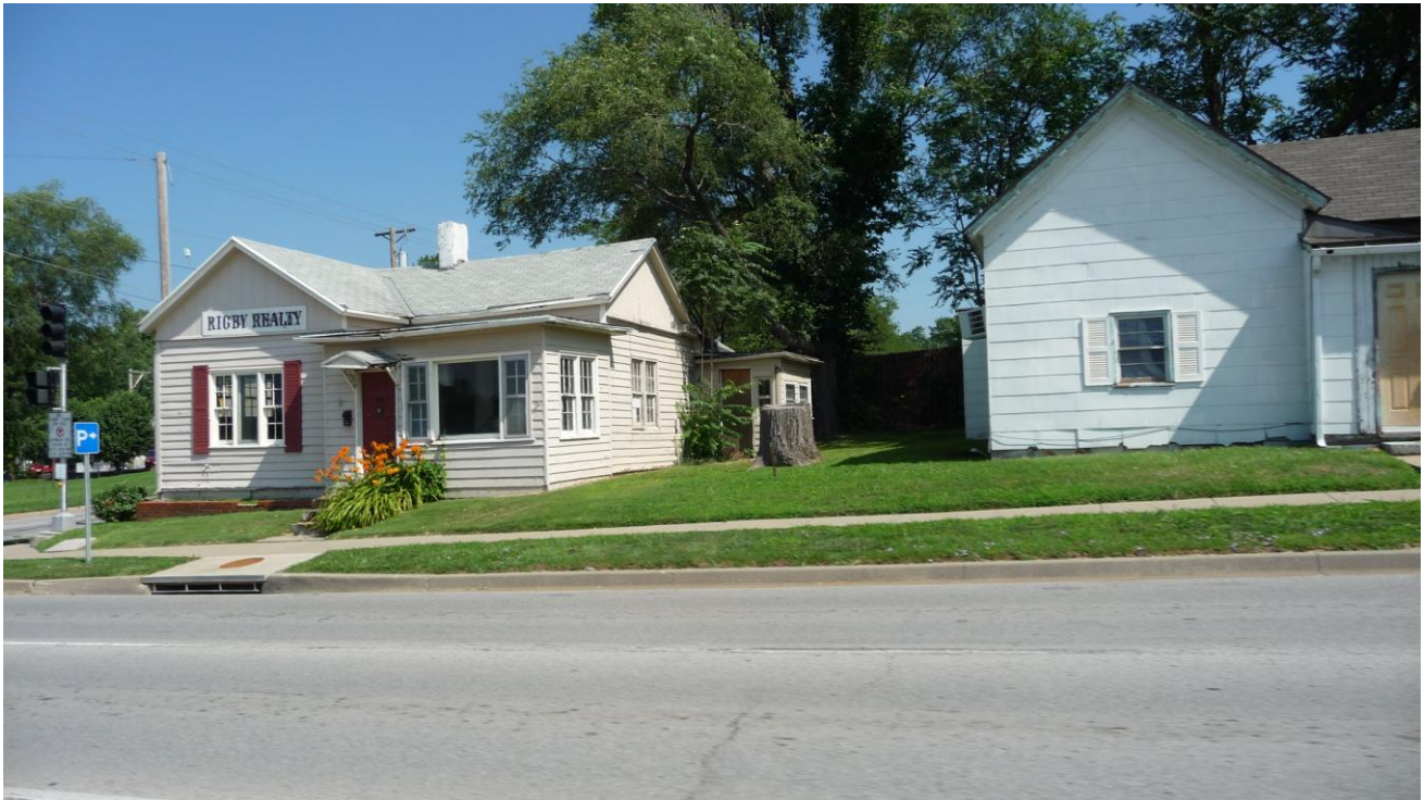
Obsolete Land-Use. 14 West Mill Street. This former single-family residence and the property to the east (10 West Mill Street) have repeated Nuisance Code Violations with the City. No improvements and continued lack of maintenance lead to structure deterioration.
