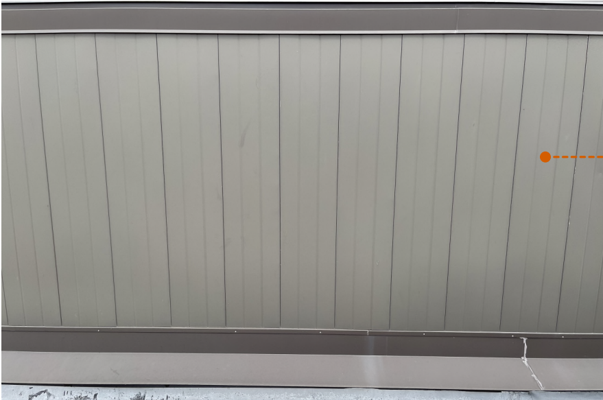
EXISTING METAL PANEL ON ROOF
