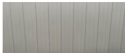
Image D: Existing metal panel on roof.
