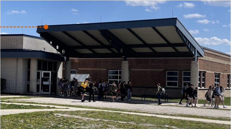
EXISTING REAR ENTRY
