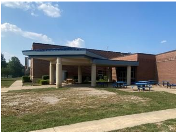
Image C: Existing blue metal roof at rear entry.
