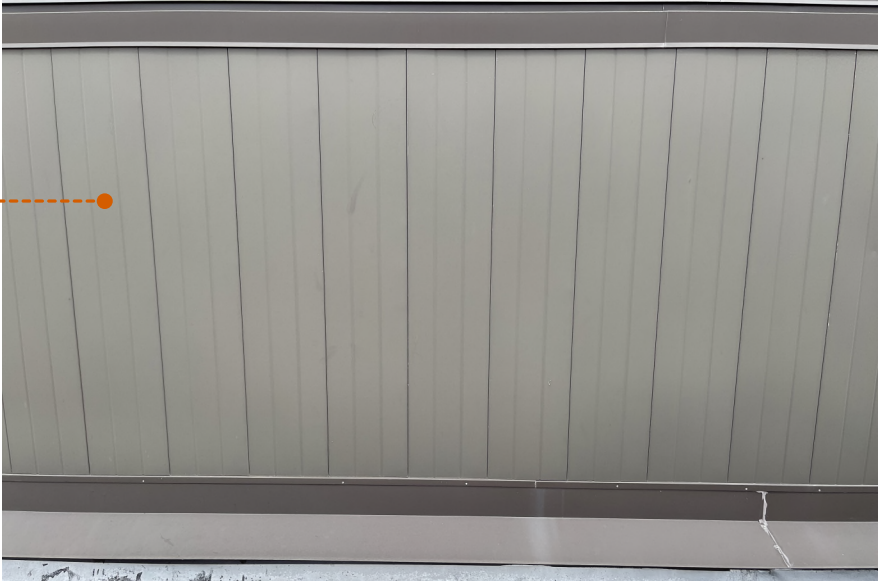
EXISTING METAL PANEL ON ROOF
