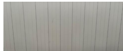
Image D: Existing metal panel on roof.
