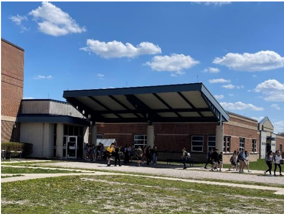
Image C: Existing blue metal roof at rear entry.
