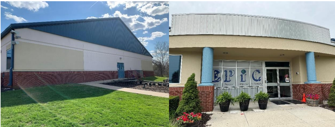
Image B & C: Existing blue and silver metal panels at EPiC Elementary.
