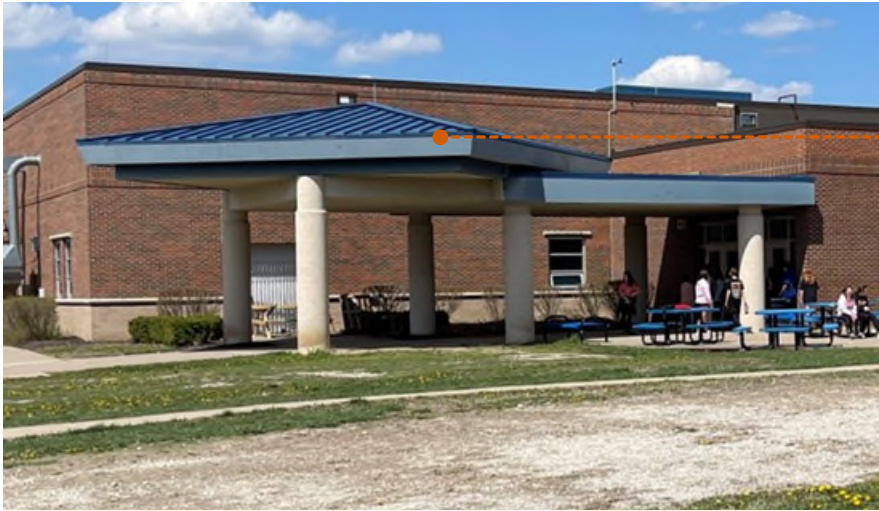
EXISTING REAR ENTRY
