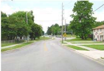
Richfield Road Today
